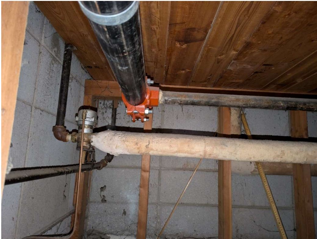
Under stage storage area – east wall near northeast corner showing one sprinkler line and hydronic piping.
