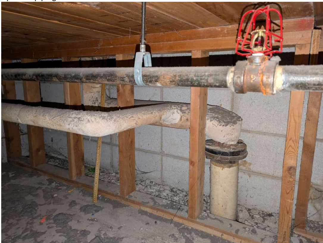
Under stage storage area – east wall near northeast corner showing one sprinkler line and hydronic piping.
